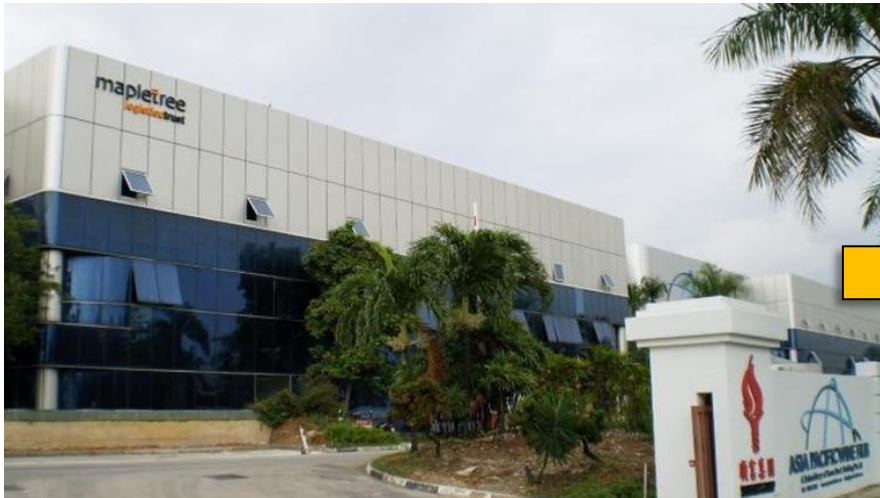
Asset before redevelopment
