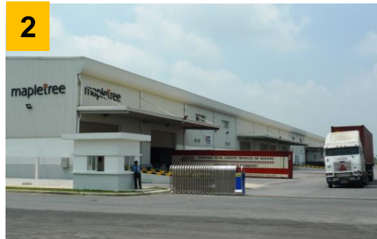
2 Mapletree Logistics Park Bac Ninh Ph 1, Vietnam
